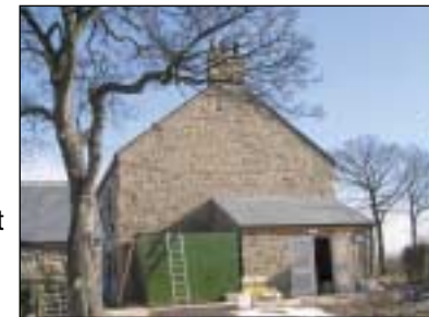
The boiler house and storage hopper at RSPB Oldmoor
