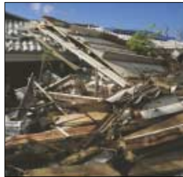
Wood waste from demolition sites
